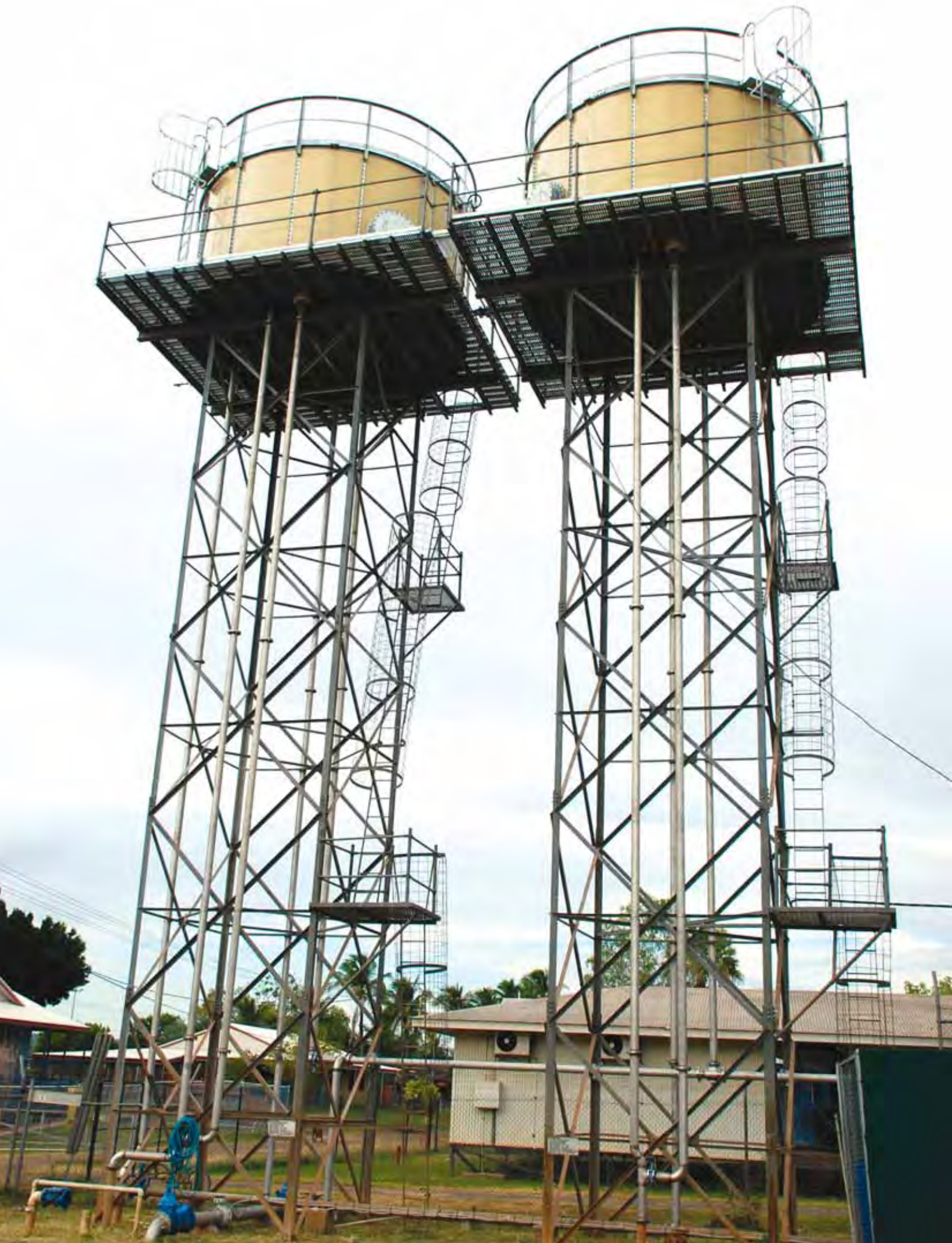
BELOW ► DALY RIVER WATER TANK
