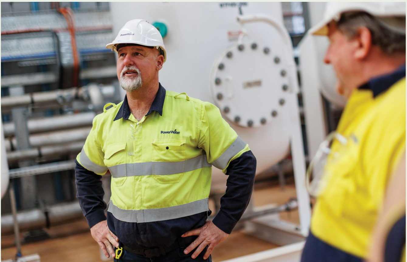
Craig Heinrich and Shawn Drewes at the PFAS water treatment plant in Katherine.
