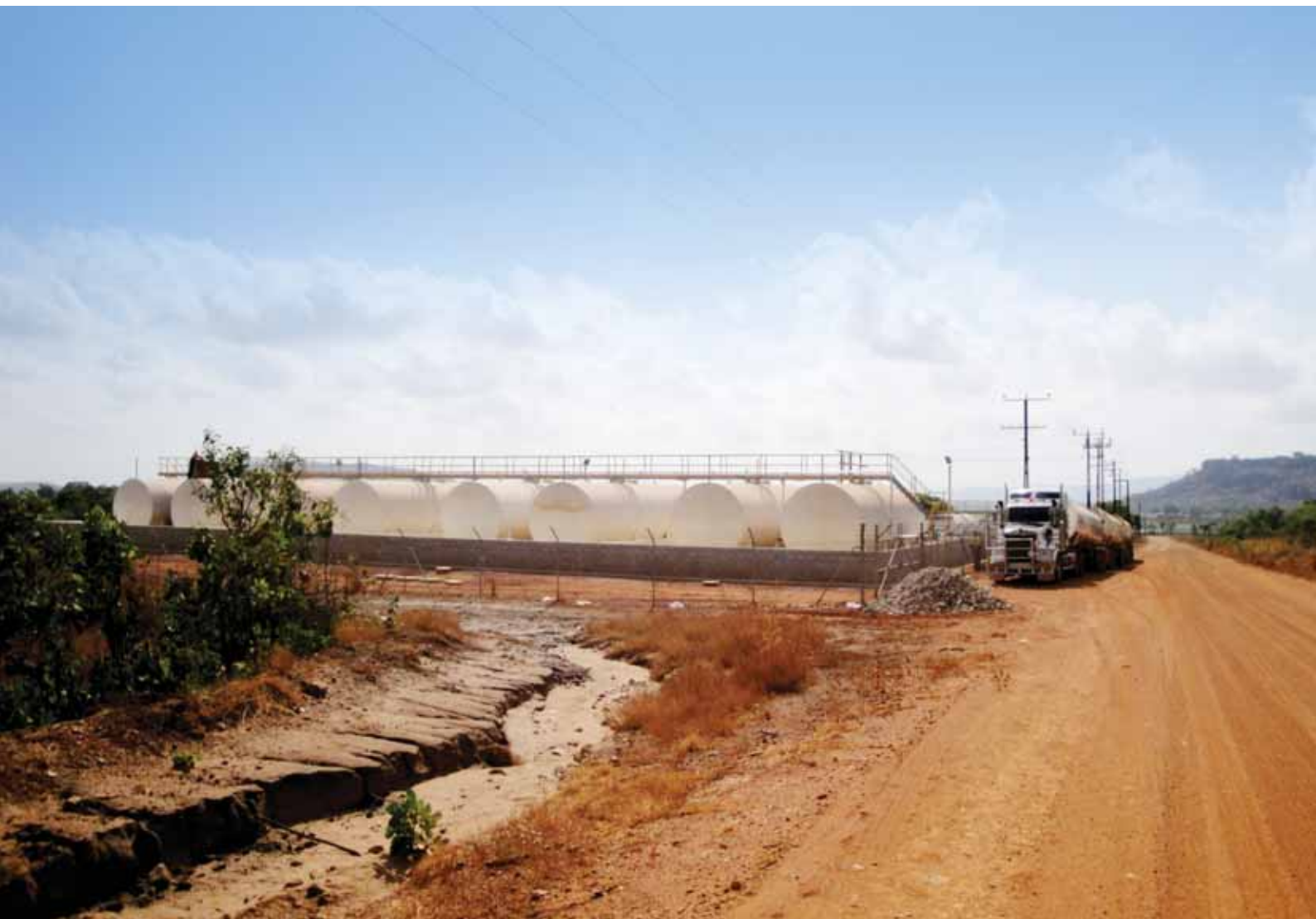
BELOW: GUNBALANYA FUEL STORAGE
