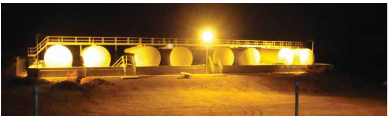
BELOW: GUNBALANYA FUEL STORAGE AT NIGHT
