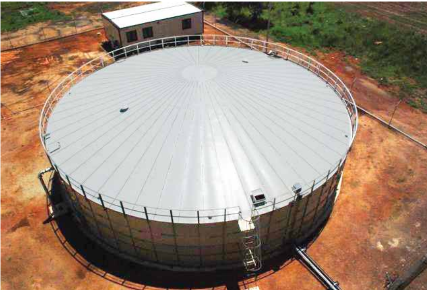
LEFT RAMINGINING TANK
