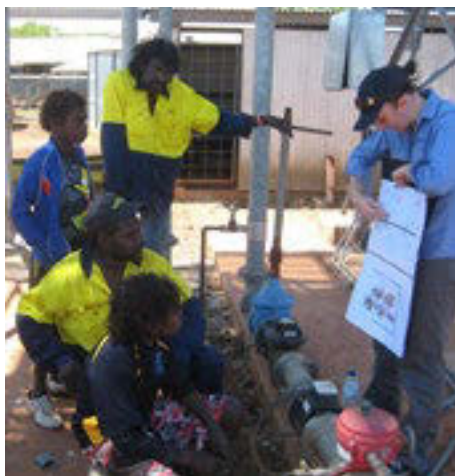
Power and Water's Kylie Climie discussing water efficiency with Minyerri residents.
