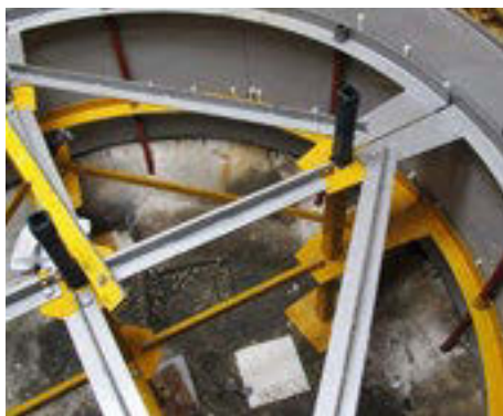
Refurbishing a sewerage pump station.
