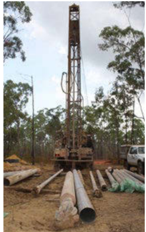
Drilling new production bores.
