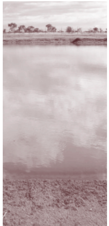
Sewer ponds at Ali Curung.
