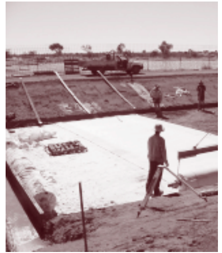
Ali Curung water and ponds under construction – installing lining.
