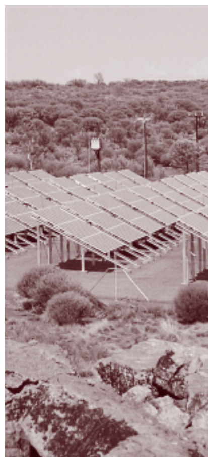
Kings Canyon, array of flat bed solar photovoltaic ponds.
