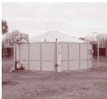
New Haasts Bluff borefield tank.
