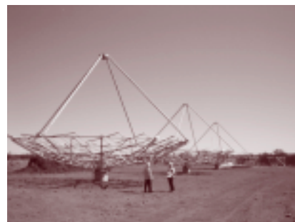
Solar dishes under construction at Hermannsburg.
