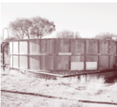
Old Haasts Bluff borefield tank.
