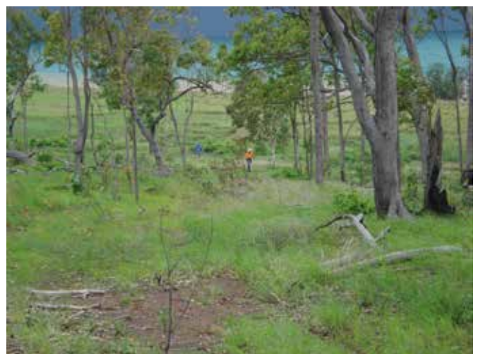
Marking out a new power-line
