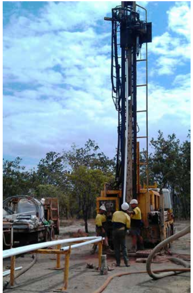
Drilling new monitoring bores
