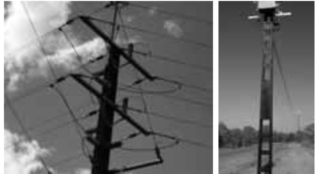
STAGE ONE CONSTRUCTION OF THE WOOLIANNA LINE
