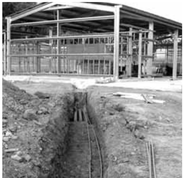
RELOCATION OF THE DALY RIVER POWER STATION
