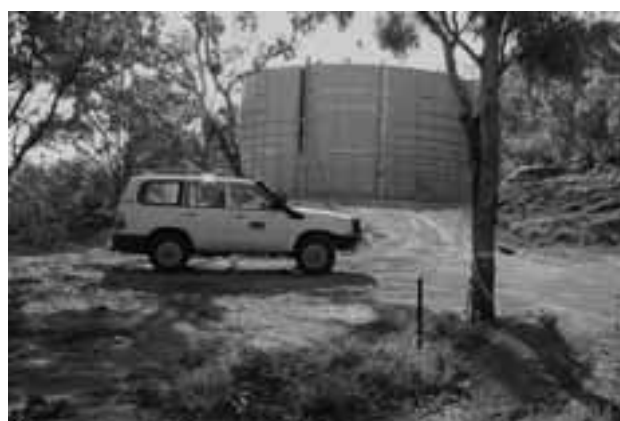
OENPELLI WATER TANK
