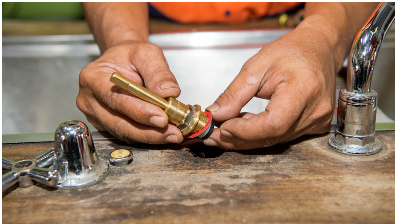
Leak checkers in Katherine helped the town save money and water.
