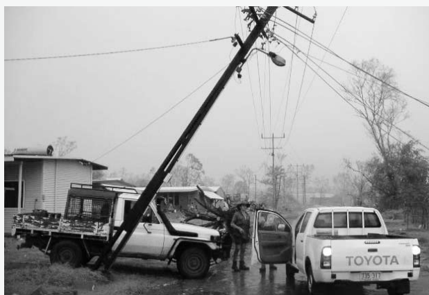
DAMAGE CAUSED BY CYCLONE MONICA.
