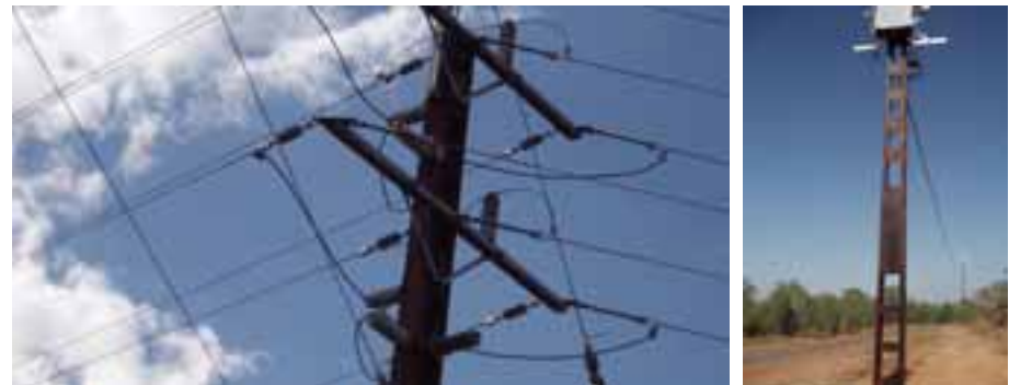
STAGE ONE CONSTRUCTION OF THE WOOLIANNA LINE
