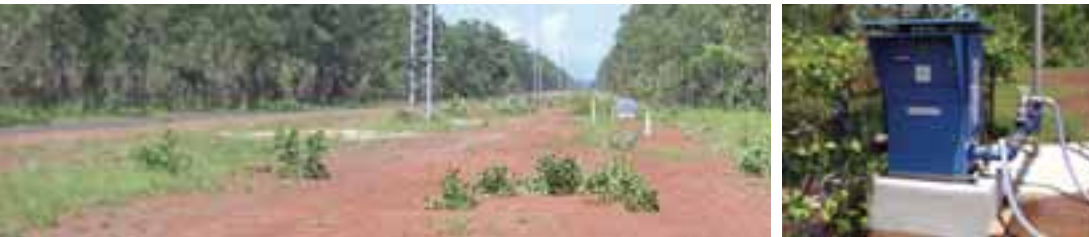
SWIPE CARD OPERATING SYSTEM AT COX PENINSULA
