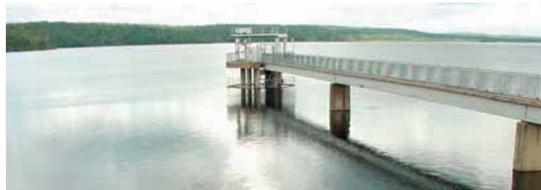
DARWIN RIVER DAM
