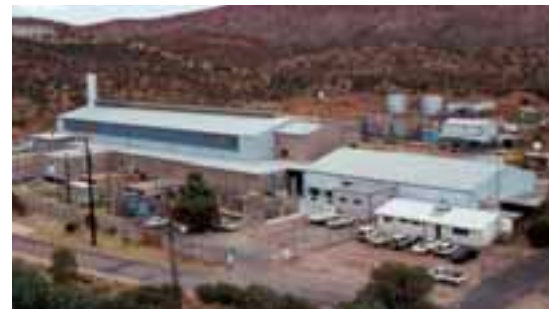
RON GOODIN POWER STATION
