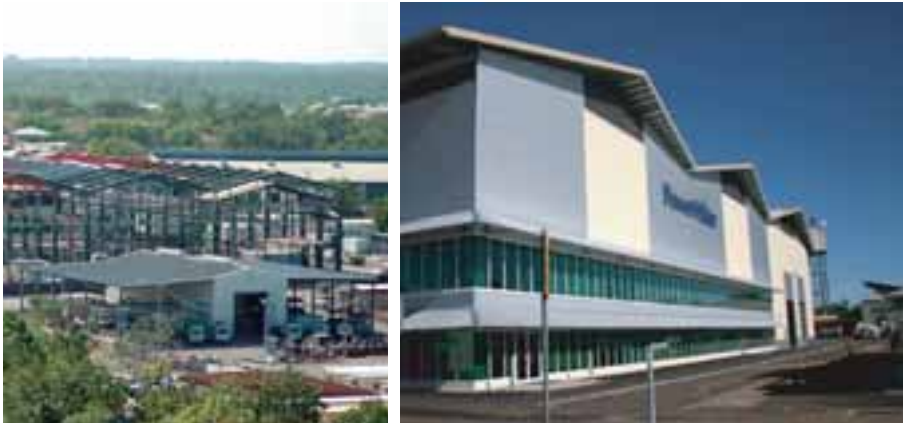
STAGE ONE OF THE BEN HAMMOND COMPLEX REFURBISHMENT
