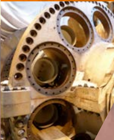
Refurbishment work on an older generation unit
