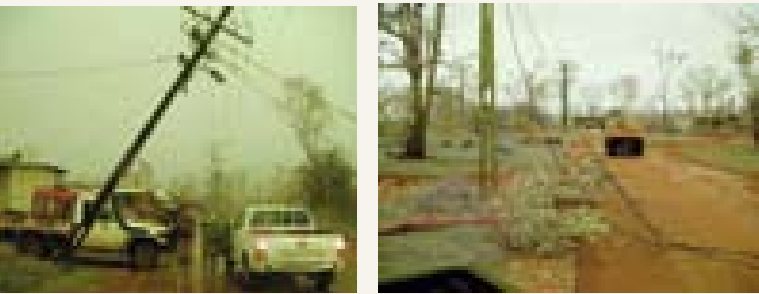
DAMAGE CAUSED BY CYCLONE MONICA.
