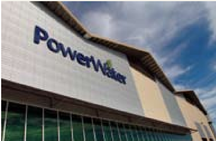
POWER AND WATER'S BEN HAMMOND COMPLEX.
