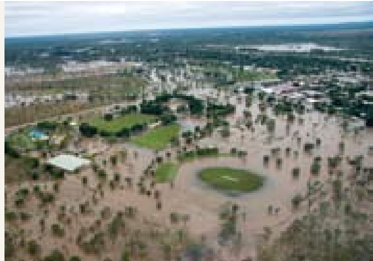
FLOODING IN KATHERINE.
