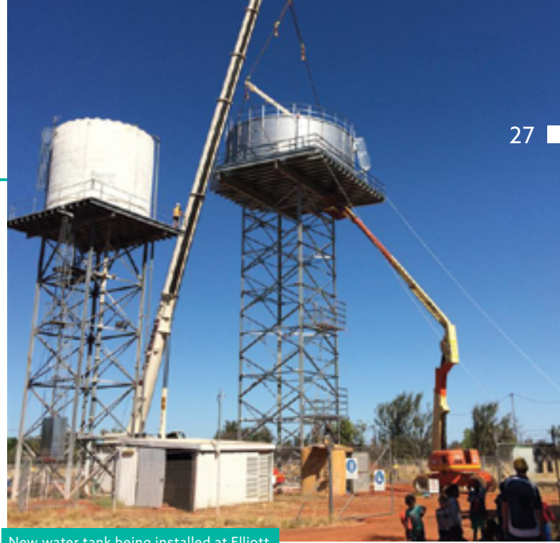
New water tank being installed at Elliott
