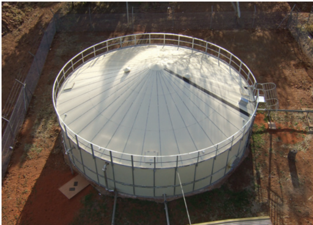
Daguragu 304 kilolitre ground level water storage tank
