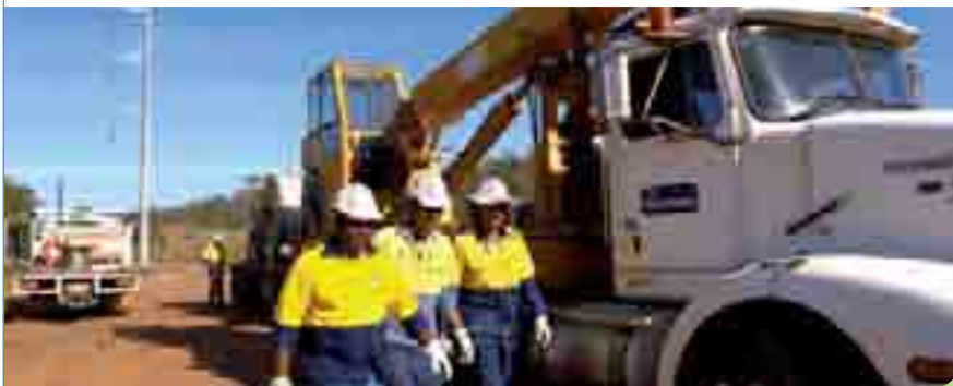
LEFT: POWER AND WATER LINE CREW AT WORK
