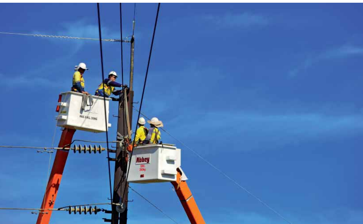
Line crews at work
