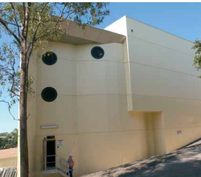
The new Frances Bay Zone Substation
