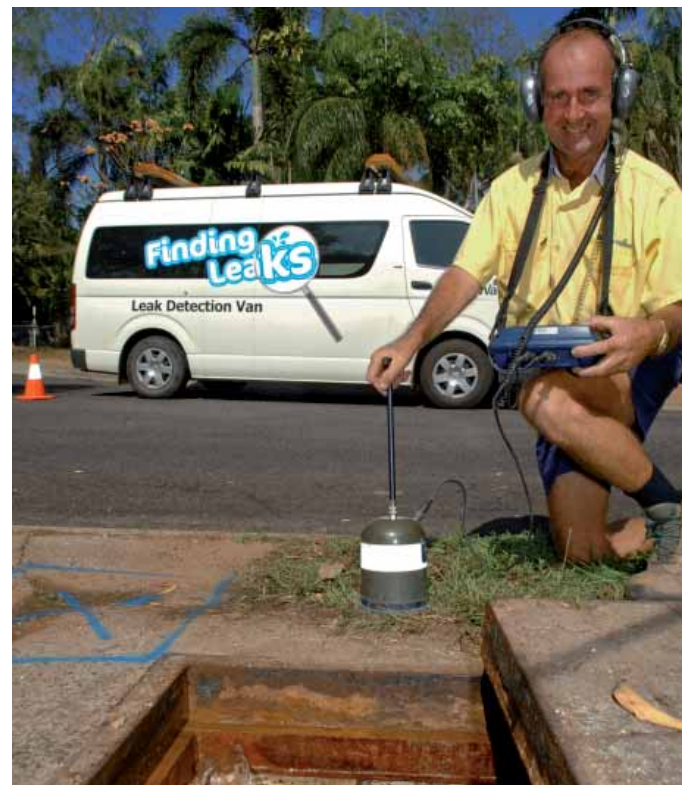
Testing for water leaks
