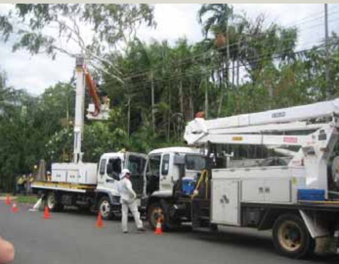
Lines crew restoring power after Cyclone Helen
