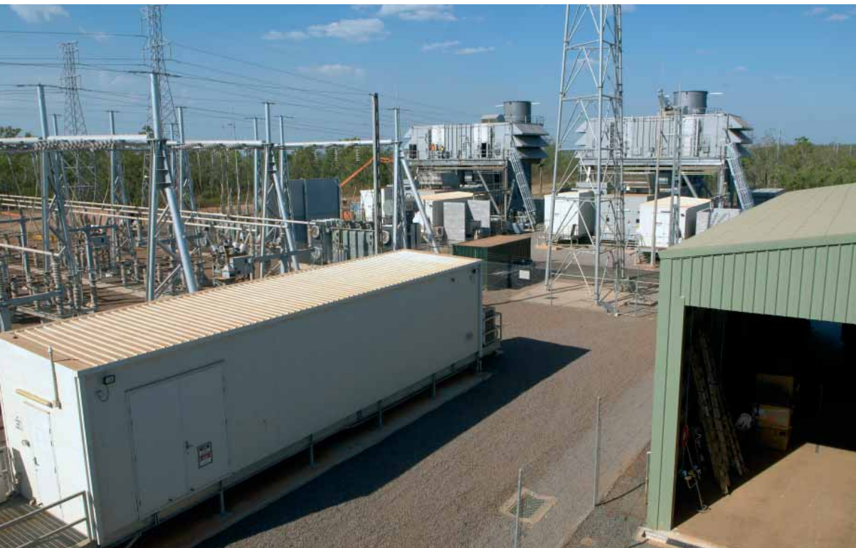
The new Weddell Power Station
