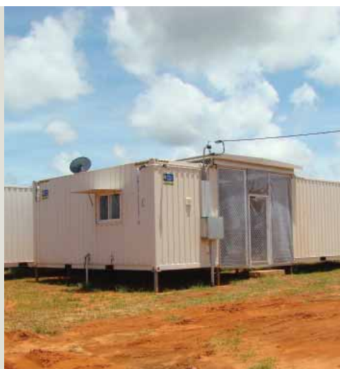
Part of the 'Vern Pechi' Maningrida Power Station
