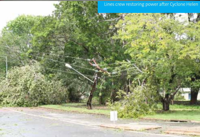
Damage to power lines caused by Cyclone Helen
