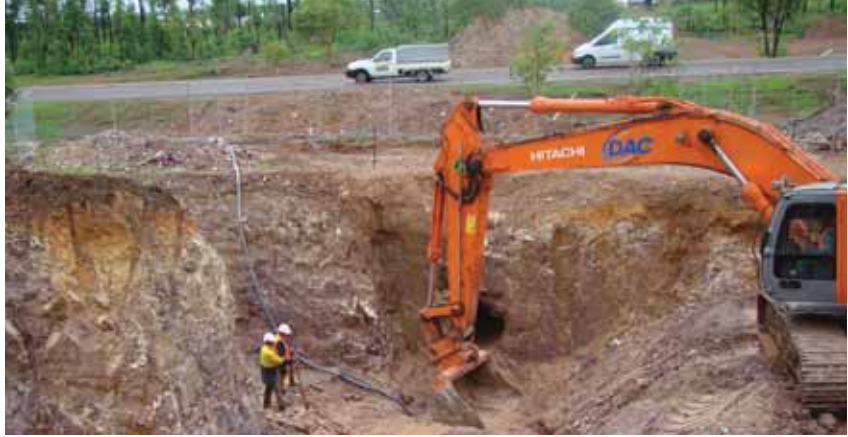
ABOVE ► THE NEW 1,000MM WATER MAIN TO PALMERSTON
