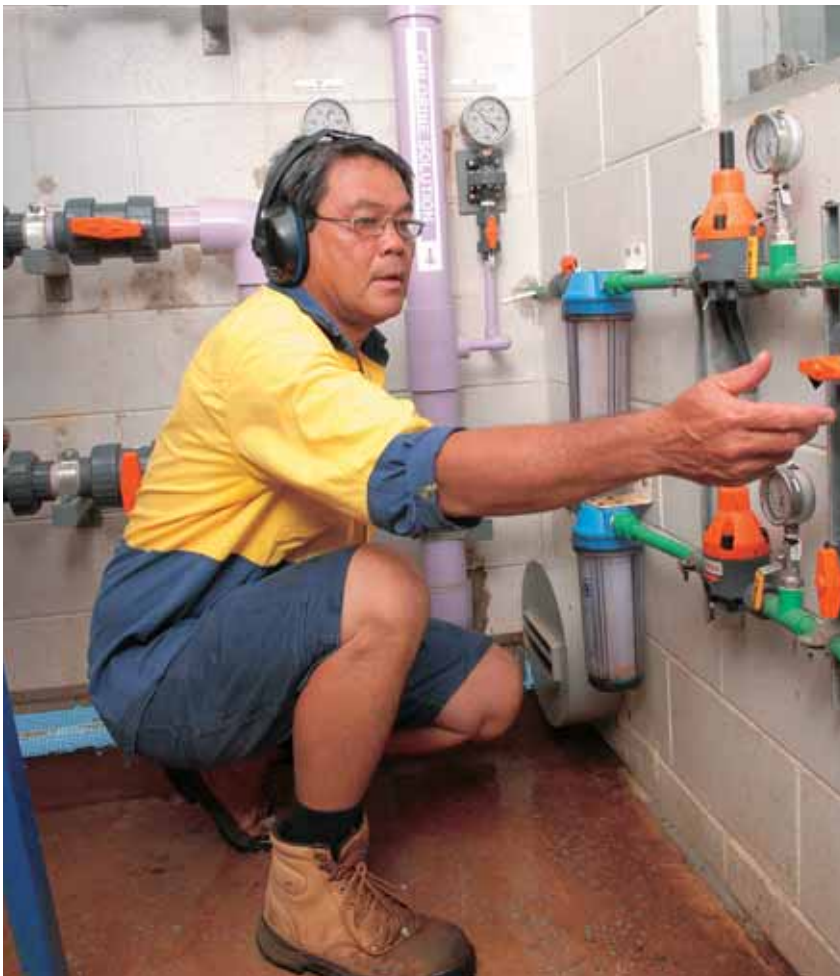
ABOVE ► WILSON LEE, WATER SERVICES AT DARWIN RIVER DAM
