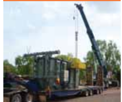
ABOVE ► A NEW TRANSFORMER BEING DELIVERED FOR SNELL ST ZONE SUBSTATION
