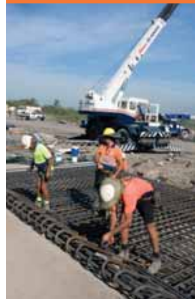
ABOVE ► PREPARING THE FOUNDATIONS OF THE NEW DARWIN RIVER DAM SPILLWAY
