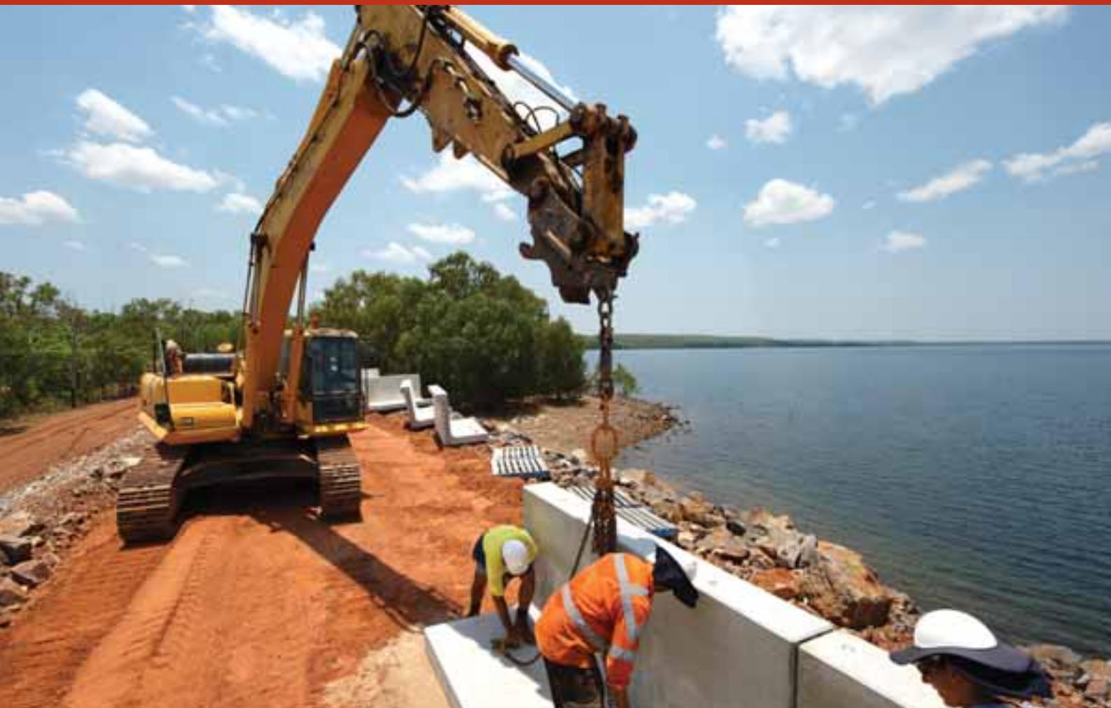
ABOVE ► RAISING THE DARWIN RIVER DAM WALL
