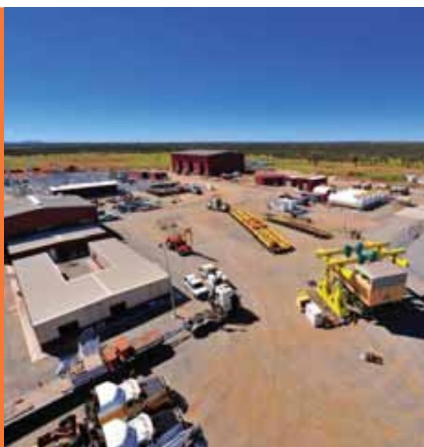
ABOVE ► THE NEW OWEN SPRINGS POWER STATION
