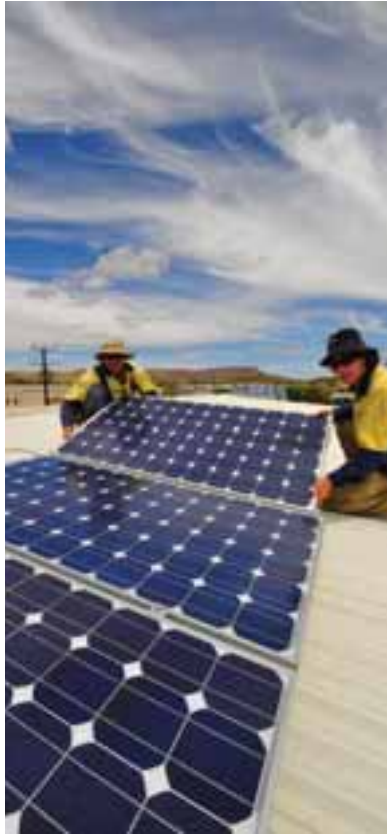
ABOVE ► A ROOFTOP PV SYSTEM BEING INSTALLED
